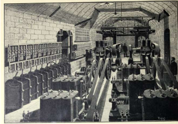
Figure 24—In the early days of electric lighting in theatres, each theatre provided its own electricity. The earliest installations employed batteries. Here is shown the power plant of the Paris Opera, as given in the
